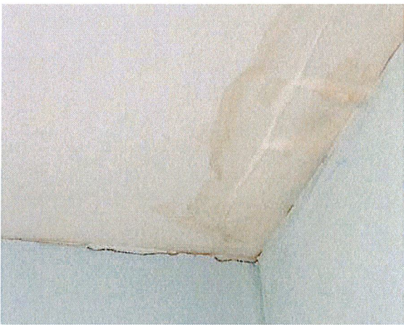
Left & Right: Interior water damage at the former convent.
