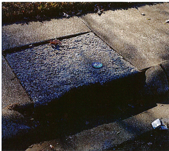
Above: A deteriorated storm drain lid located along South Metter Street.
