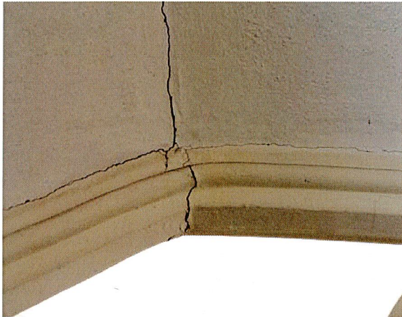
Left: Cracking in an archway inside the vacant church.
