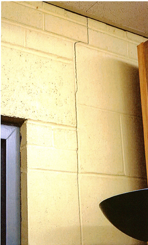
Left: Cracking in the concrete block wall inside of the former rectory.
