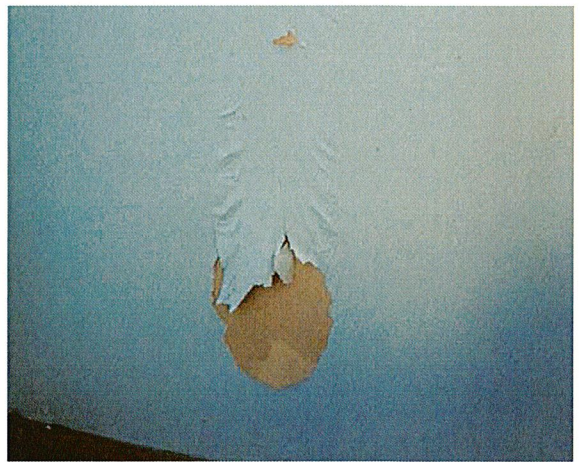
Left & Right: Interior water damage at the former convent.
