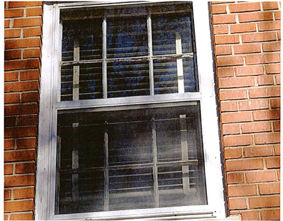
Left & Right: The windows on the former convent are deteriorated and need to be replaced.
