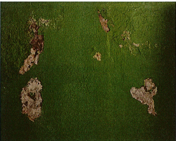
Left: The concrete on the interior basement walls is spalling.
