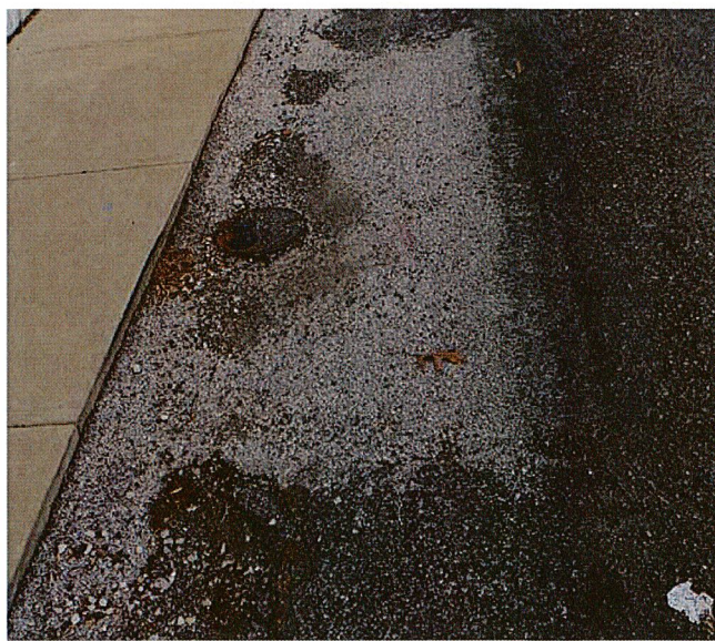
Above: The edge of the pavement along West Washington Street is deteriorated. (December 15, 2015)
