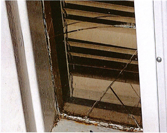
Left: The side-lite windows on the rectory are cracked.
