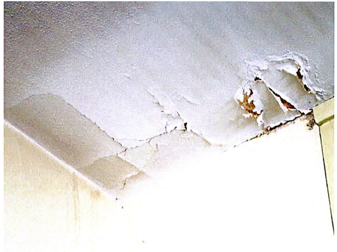
Above & Below: Interior water damage of the vacant church.
