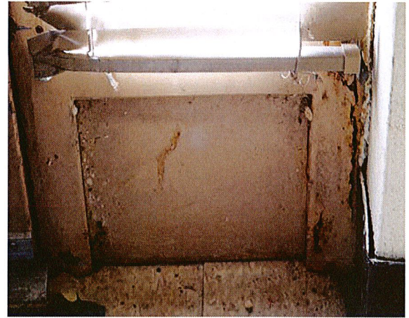
Right: The metal frame under the side lite of the rectory has rusted.
