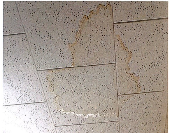
Right: Interior water damage to the ceiling tiles inside of the former rectory.
