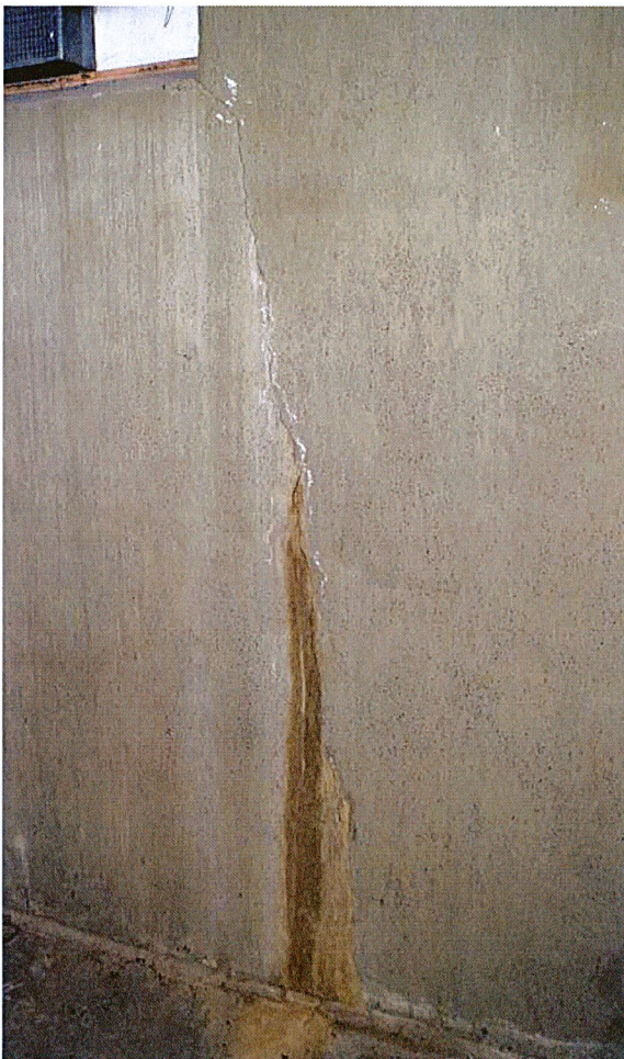
Left: A below grade crack in the basement foundation of the former rectory allowing water to infiltrate the structure.
