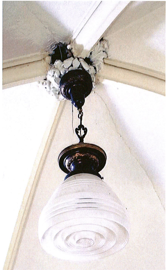
Right: The medal- lion supporting the light fixture in the church has detached from the ceiling, leaving the fixture hanging.
