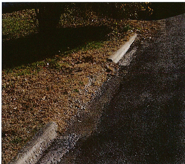
Above: A missing curb and deteriorated edge of pavement along South Metter Street.
