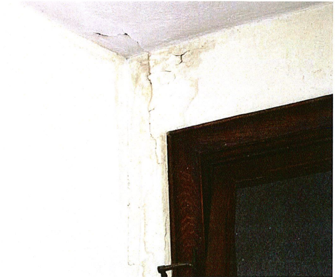
Above & Below: Interior water damage of the vacant church.
