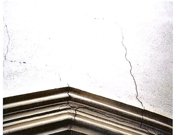
Left & Right: Cracking in the plaster and mold- ing of the church ceiling.
