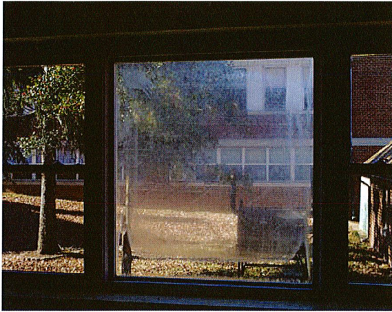
Left: Moisture in the window of the former rectory due to a broken seal.
