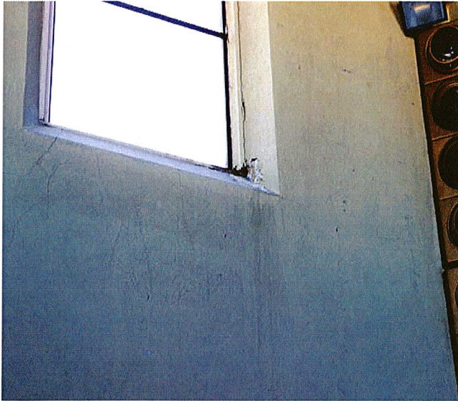
Above: The rotted window frame and deteriorated plaster at the corner of this window indicate interior water infiltration.
